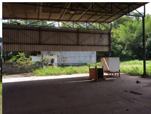
Pipe-shop (vista interna)
