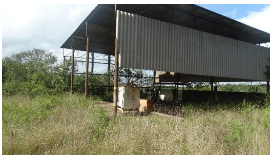
Pipe-shop (vista lateral) : 300m2
